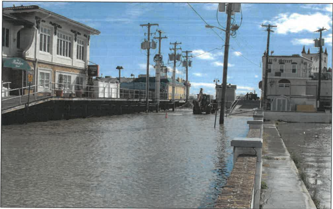
Flooding on 11th Street, Ocean City, NJ
