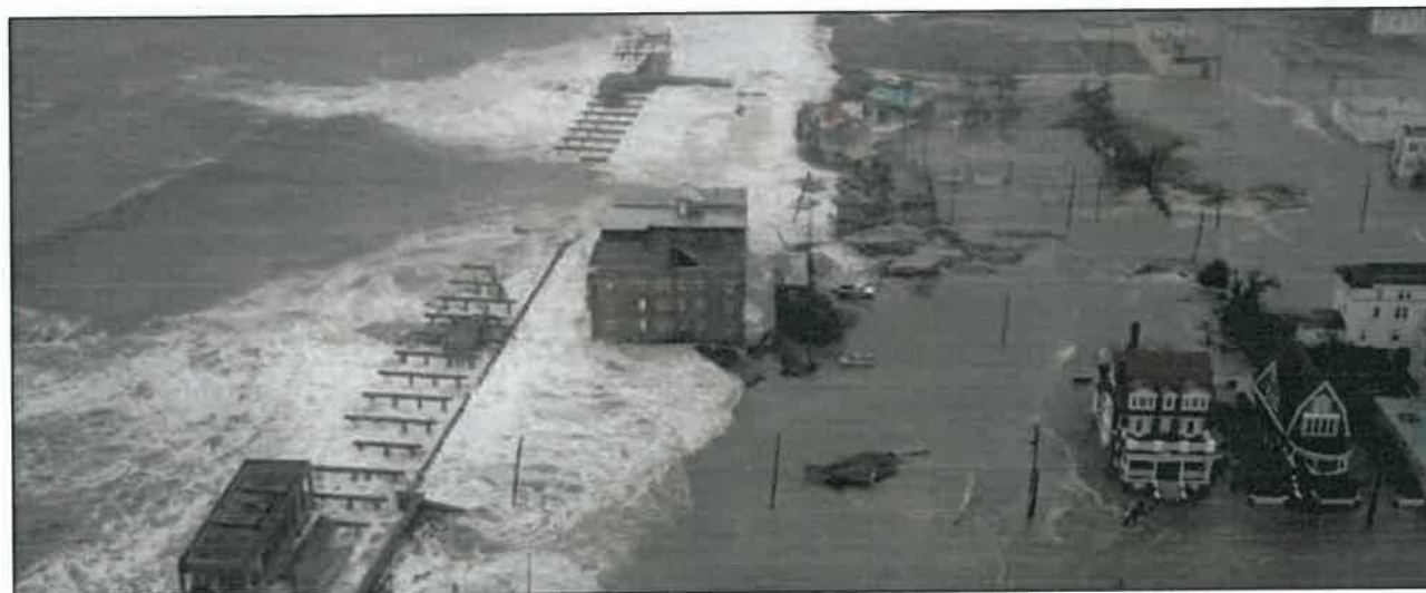
Inlet Section of Atlantic City, NJ after Hurricane Sandy
